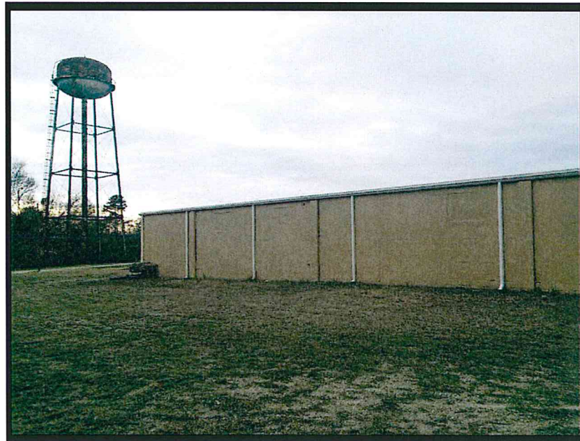
Southwest view from site (Main Street Site)
